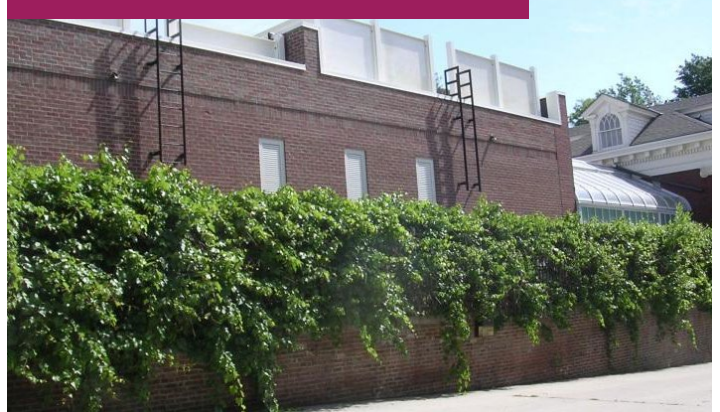
Architectural Screening - Roof Mounted
